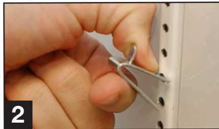
2 (Installing bottom of the shelf clip)
